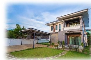
5 Lines Prime property (€750,000)
